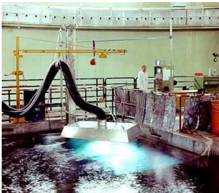
Figure 4. Underwater plasma arc cutting in operation
