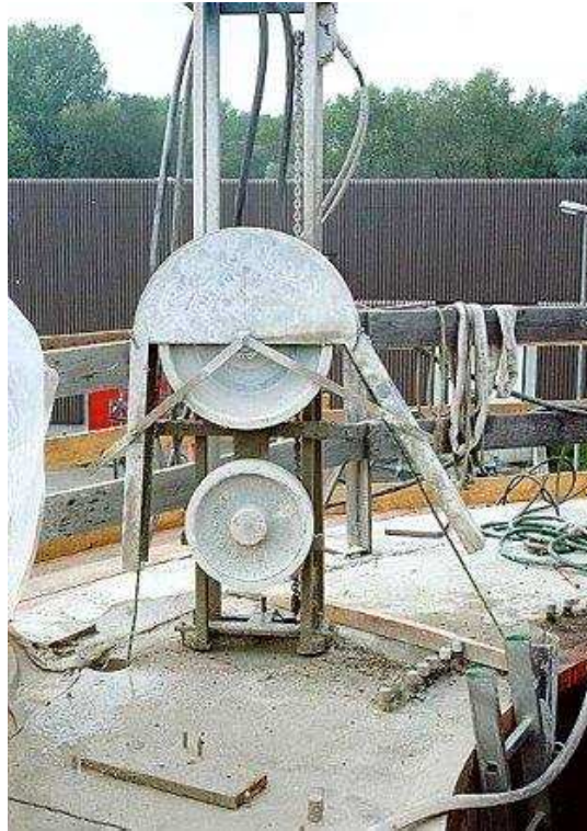
Figure 33. Diamond cable cutting equipment at the bio-shield mock-up
