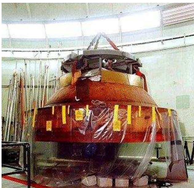
Figure 2. The RPV-cover after lifting from the vessel
