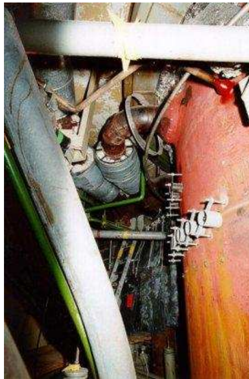
Figure 27. Situation in the upper circular room, above the bio-shield
